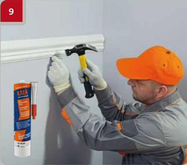
If using G06M290 adhesive it is necessary to hold it with finishing nails hammered under the product to prevent the product from sliding. The nails are removed after 24 hours.
