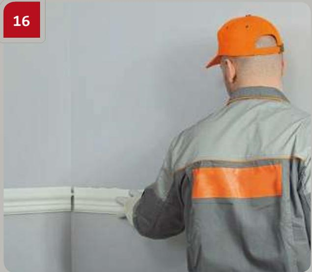
Press the product to the wall so that adhesive exudes from under the whole surface of junction. While moving the product along the wall, push it to the adjacent product so that adhesive exudes from the joint.
