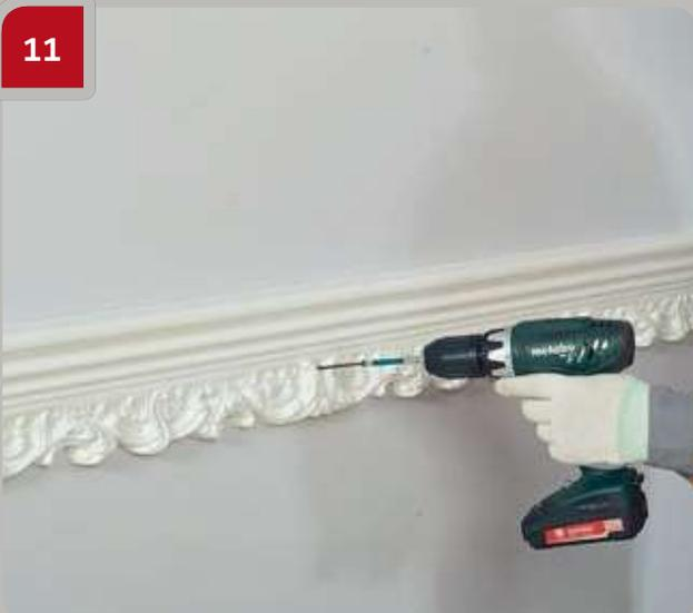
For products of more than 100 mm height, additional fixation with self-tapping screws at a spacing of about 600 mm is required.
