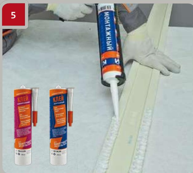
Apply G06M290 adhesive on the mounting surface or G10U290 adhesive along the length of the product. The thickness of the applied layer of adhesive shall be 3-5 mm.
